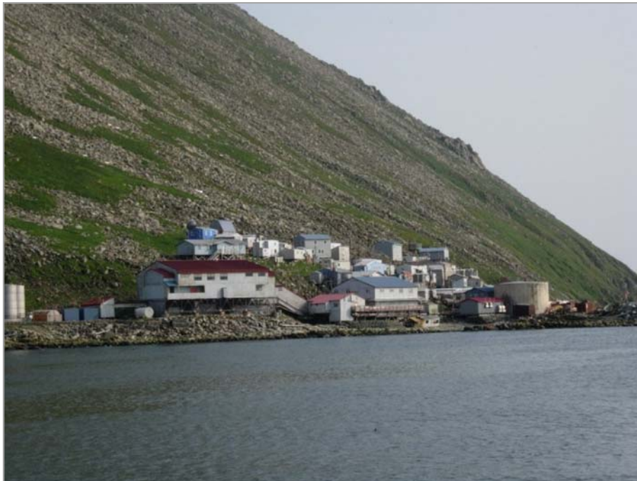
Little Diomed School Renovation
