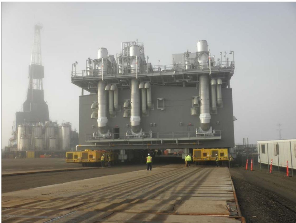
ENI Utility Module Offload
