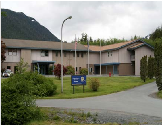
Department of Public Safety Academy
