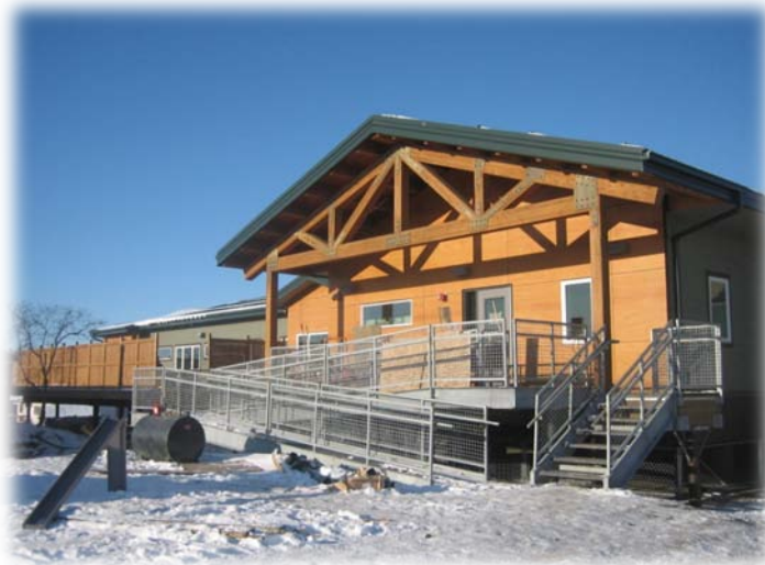
Tundra Women's Coalition (TWC) Bethel. TWC's recently completed shelter facility.
