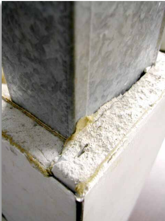
The gypsum-wallboard covered steel stud is only part of a fire-resistive rated assembly.
