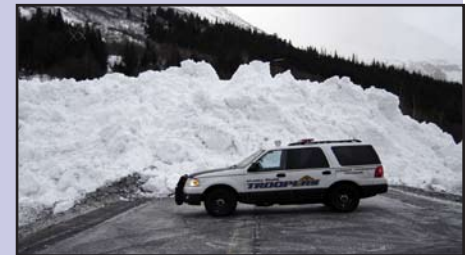
Trp. Dan Cox snapped this photo of an avalanche across the Seward Highway at about 21 mile. The avalanche crossed the highway and railroad with debris stretched all the way to the Kenai Lake, blocking off the flow of traffic and the railroad on Feb. 19, 2008. The road was closed for 20 hours while DOT cleaned up the snow.
