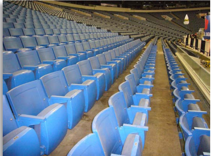
Aisle width for this large assembly occupancy is determined by the number of seats in the row.
