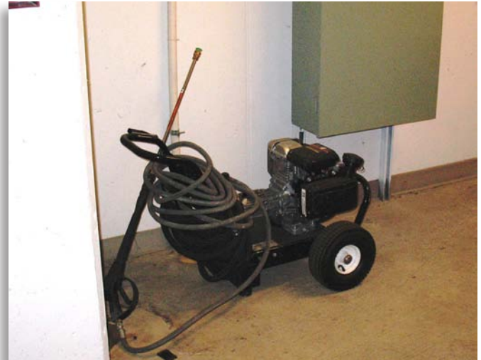
This gasoline-powered pressure washer may be allowed indoors under certain conditions, but should be kept away from the electrical service. Photo contributed by Byron Blake.
