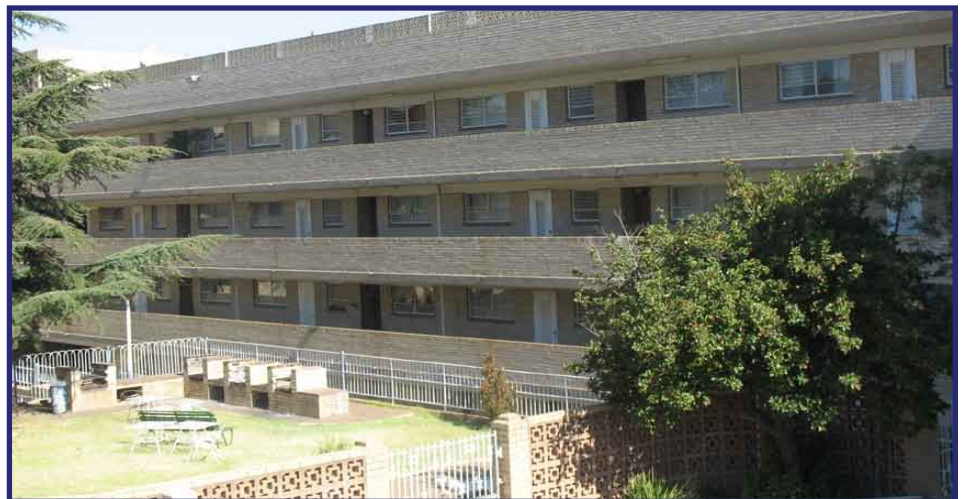
A housing unit at the Fairview fire station in the Inner City district of Johannesburg. As a safety measure most of the fire stations are surrounded by security fences and high walls.
