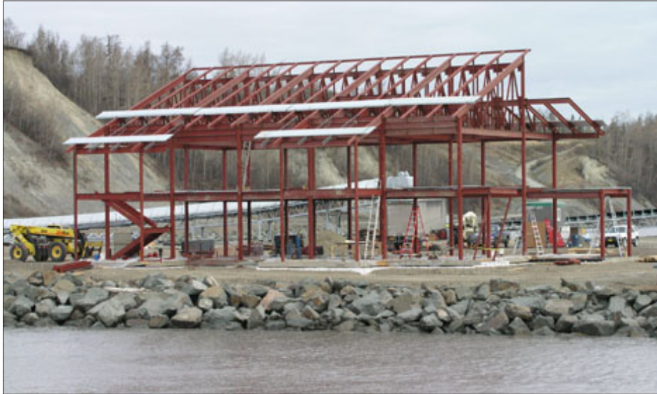
A new ferry terminal is now under construction at Point McKenzie.
