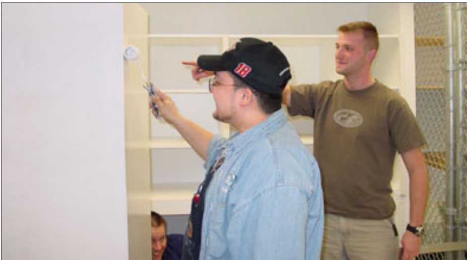
PV Enforcer Vessel Tech II Ray Streitmatter and Public Safety Tech Charlie Johnson putting the finishing touches on the Evidence Room storage shelves.
