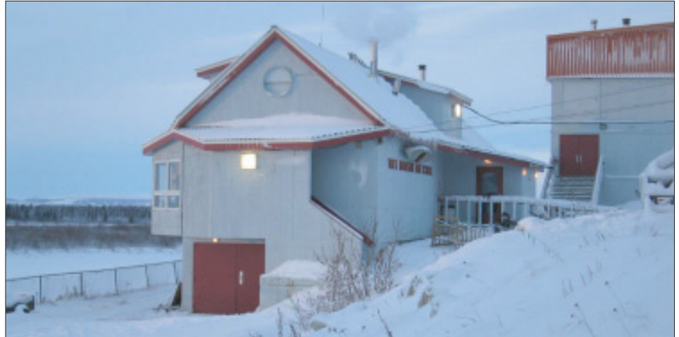
White Mountain School before the fire.
