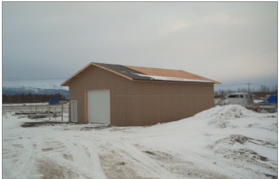
The new ABWE Palmer Shop was built with much hard work by Fish and Wildlife Aides Jaime Kirkmeyer and John Ekelmann. Their skilled work significantly reduced the building costs. The shop will be used to store and maintain ATVs and boats.
