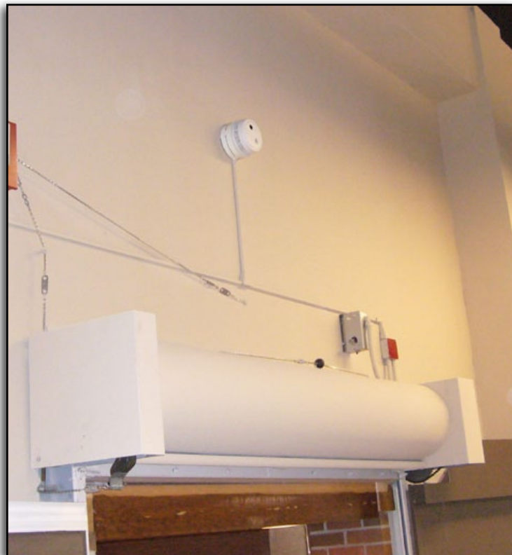
Fusible links to release this opening protective should be located near the ceiling.
