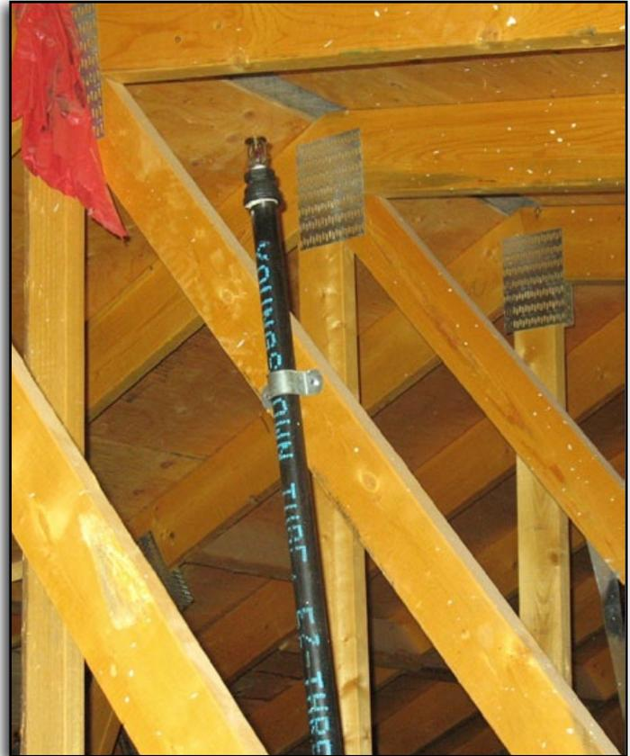
Photo courtesy of Freedom Fire Protection, LLC, Longmont, Colorado. Because of its length, this sprig must be supported to restrain lateral movement.
