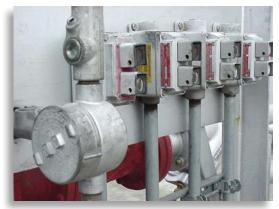
These explosion-proof switches are installed in an environment where flammable vapors are present.
