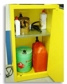
This flammable liquid cabinet is designed and built in accordance with Underwriters Laboratories (UL) 1275, Flammable Liquid Storage Cabinets.
