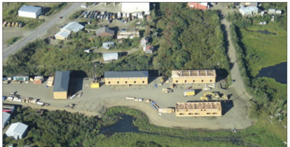
An aerial view of Bethel's new post photographed by Sgt. Perry Barr.
