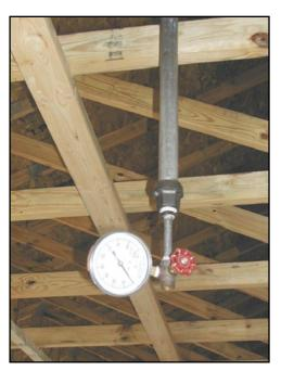
Sprinkler hydrostatic tests are measured at the lowest point of the system or portion of work.
