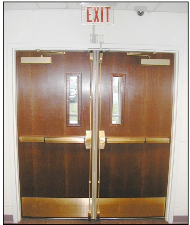
This pair of exit doors is just one part of the overall means of egress.
